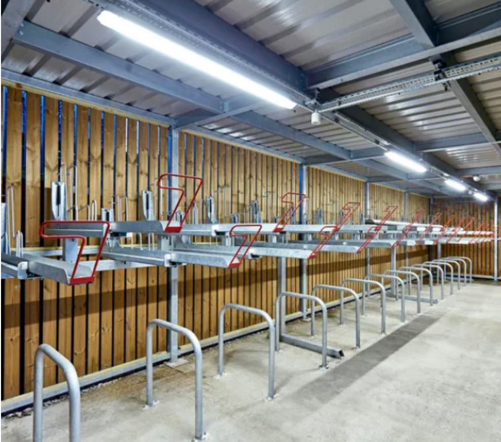
EXAMPLE OF STACKING SYSTEM PROPOSED WITH SHEFFIELD STANDS AT LOW LEVEL AND STACKING SYSTEM ABOVE
